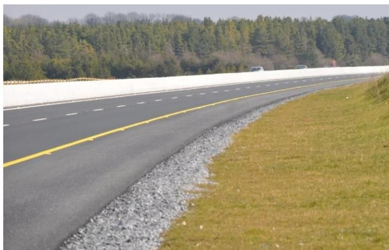
**Figure 6.7 Example Filter Drain**
