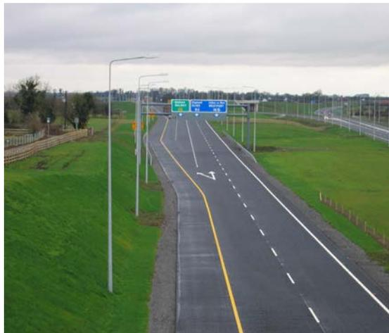
**Photo 3.6.9 Filter Drain on M4 Motorway**
