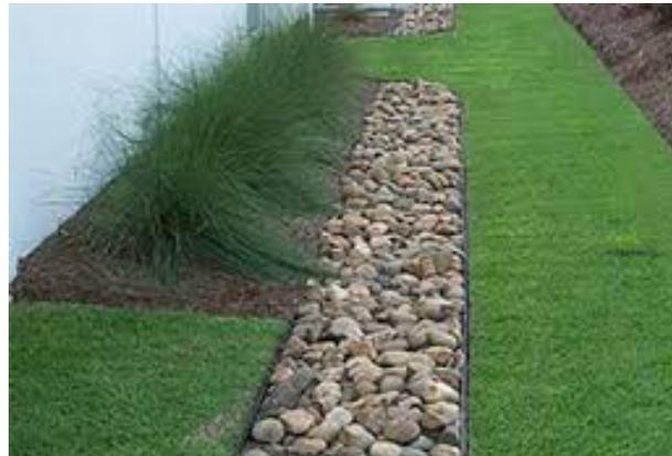
**Photo 3.6.7 Infiltration trenches/ soakaways**
