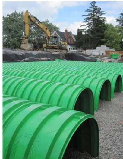
**Photo 3.7.4 A Triton™ Subsurface Attenuation System (source: [www. http://terrafixgeo.com](http://terrafixgeo.com) )**
