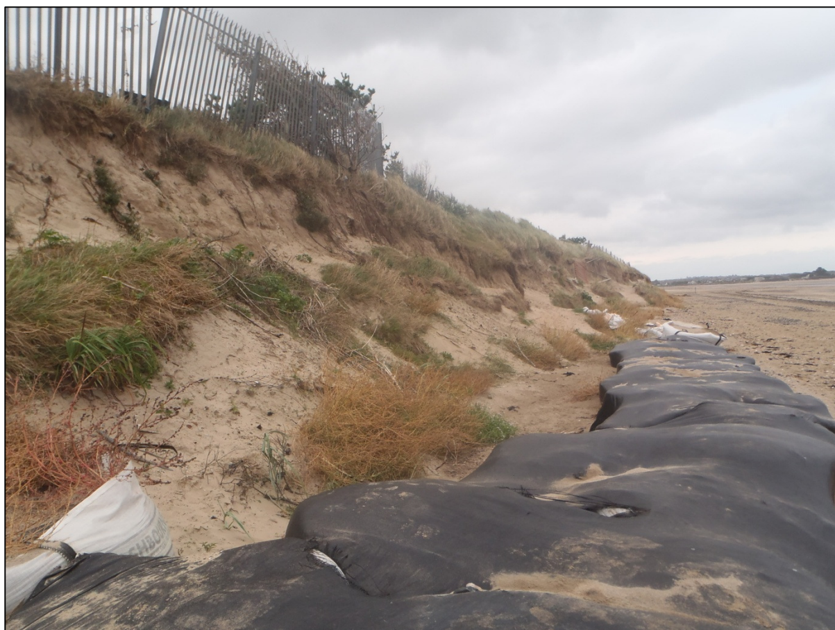
Figure 8. Location of the proposed buried rock revetment. Covered sand bags are visible in the foreground, with a narrow strip of 1210 Drift line vegetation found landward of these.
