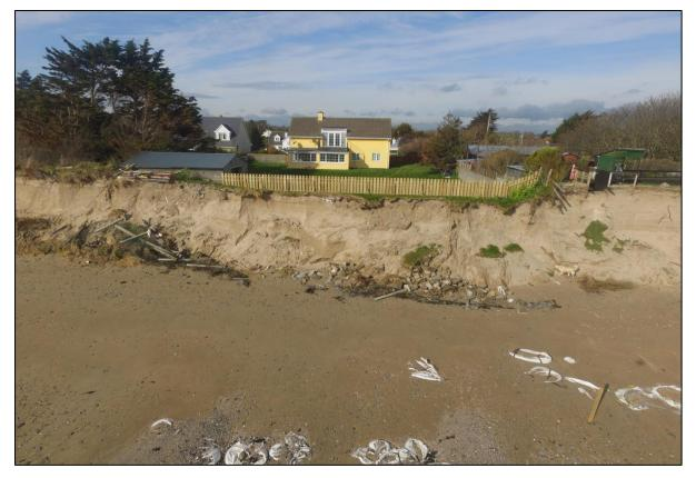
Figure 4.2: The severely eroded dune system and debris in front of residential property E.
