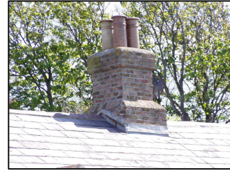
Fig. 10 Chimney stacks & pots
