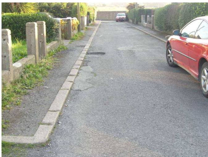
Fig. 5: Street surface and boundary to front gardens
