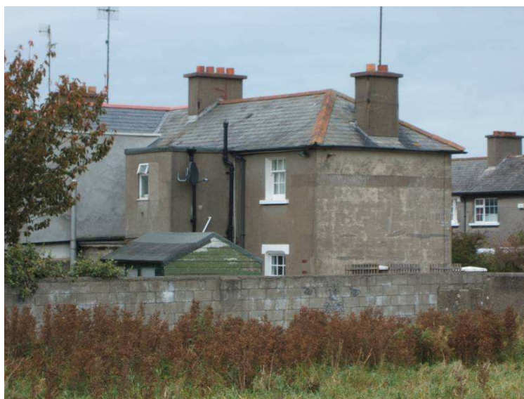
Fig 15: View of end of terrace situation to south-west
