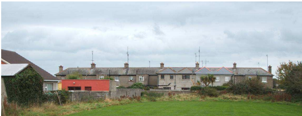
Fig 13: View of the rear of the western terrace
