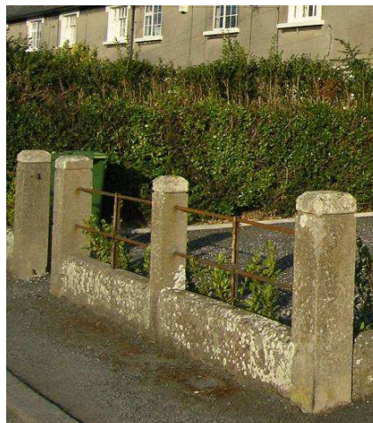
Fig. 6: Original railing at house number 54
