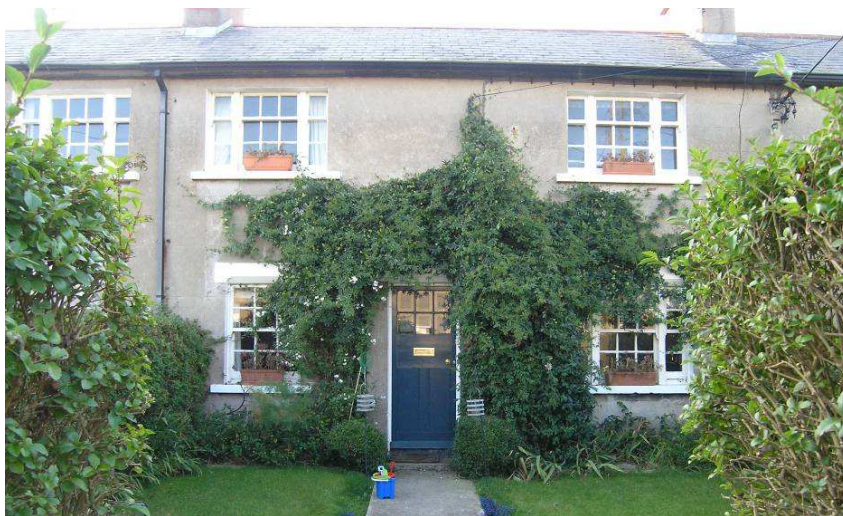
Fig. 8: House no. 56 with original front door and windows
