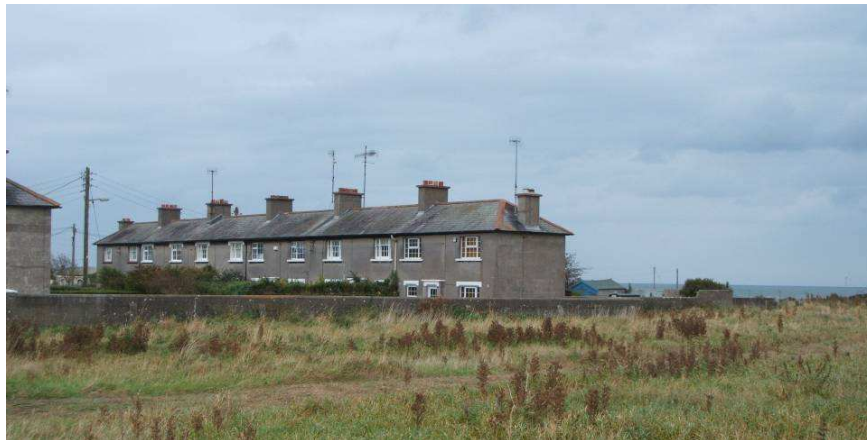
Fig. 19: View of The Grey Square from the south in the direction of the sea
