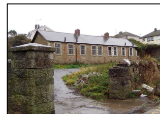
Fig. 15 Former National School, Balglass Road
