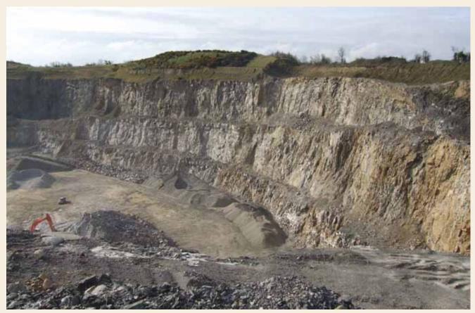
A view into part of Feltrim Quarry from the rim. Although Feltrim Hill is slightly higher than surrounding land, the quarry has been excavated to some depth below the general level. Quarrying is done in stepped benches for stability and safety of the faces
