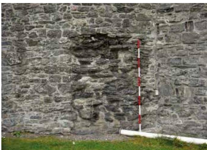
**PLATE 46:** Restored wall showing original fabric
