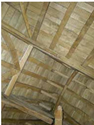
**PLATE 58:** *Constable's Tower interior, top floor. View of new roof trusses and boarding*
