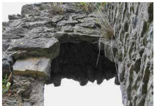
**PLATES 38 AND 39:** *View to doorway between the Archbishop's Apartments and the East Tower (left); Close-up of the 'Caernarfon arch' over the doorway (right)*
