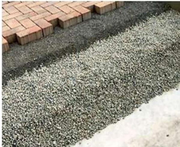
Typical Permeable Paving
