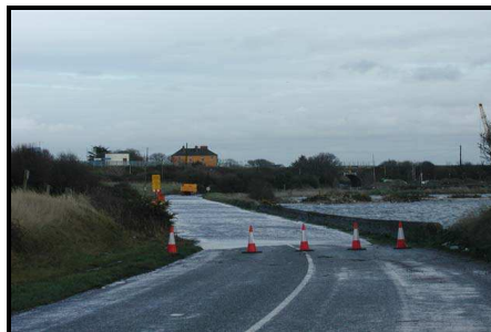
Tidal flooding at Laytown, Feb 2002
