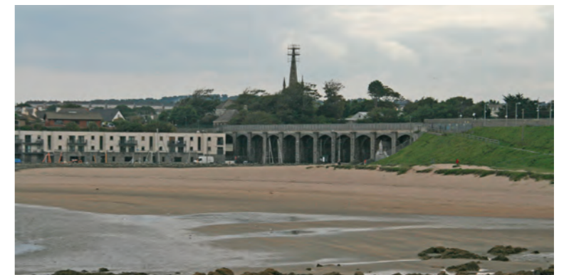
Beach and Railway Viaduct
