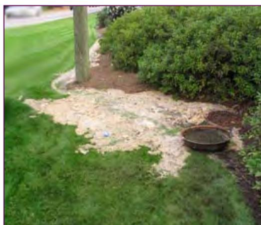
*Photographs 1 and 2 show overflows caused from FOG blockages in the sewer.*
