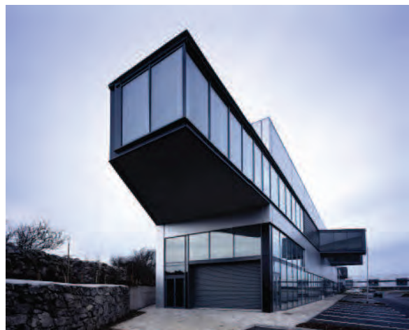
Image 4.8: High Architectural Quality Business Park Building
