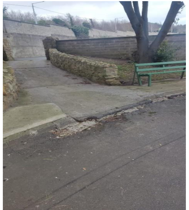
Concrete and macadam repairs at St Fintan's burial grounds ongoing.
