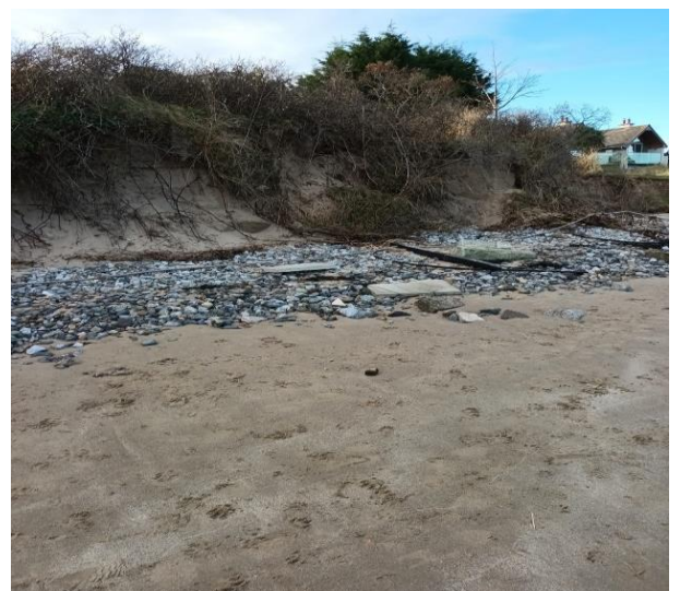
Ongoing repairs to our dune protection posts and ropes Burrow Beach Howth.
