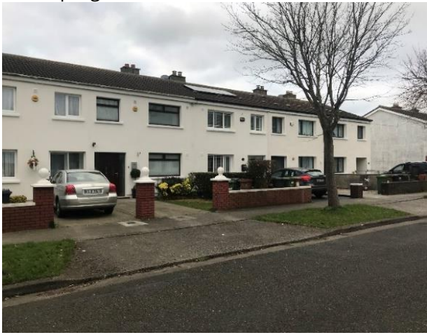
Post-works – Strandmill Estate, Portmarnock (external wall insulation, new windows and doors)
