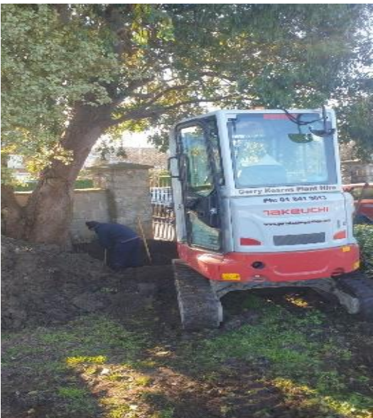
Repair of water leak at Balgriffin burial grounds
