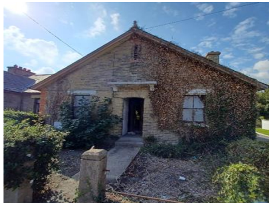
Derelict Property 73 Portrane Ave. St Ita's
