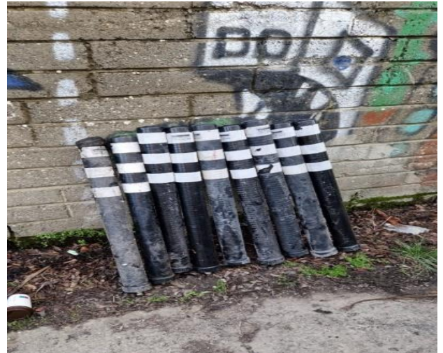
Removal and replacement of cycle lane bollards Howth Malahide areas.
