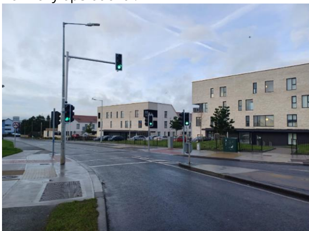
New signalised pedestrian crossing on Church Road
