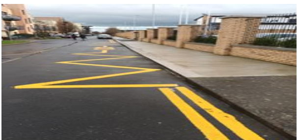
Stapolin School ETNS - New line marking commenced across road frontage
