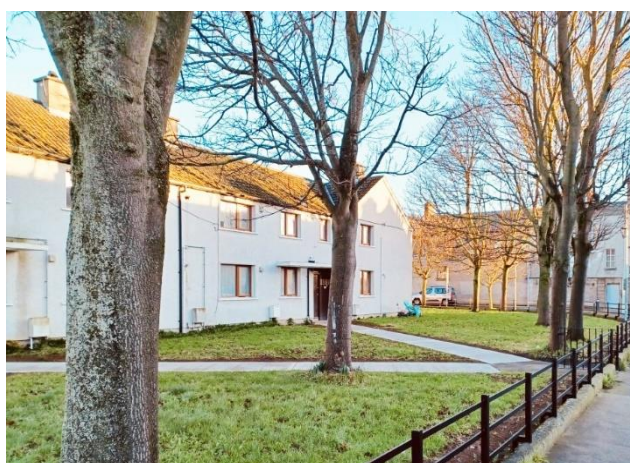
Dublin St Flats, Baldoyle - Front Area
