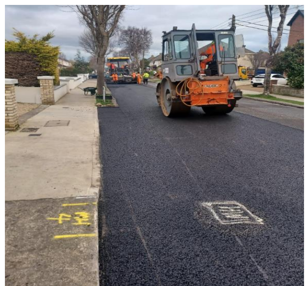
Wearing course being laid on Texas Lane during Road Inlay
