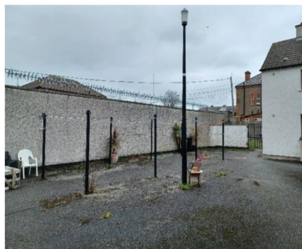
1 Rear Area/Yard - Before Upgrade
