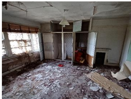
Example - Room Before Renovation
