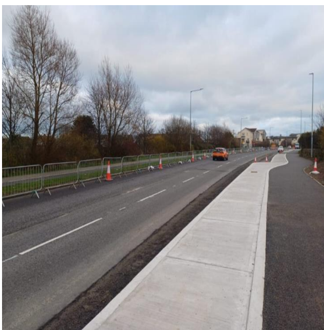
Works completed on the south side of the Hamilton Road
