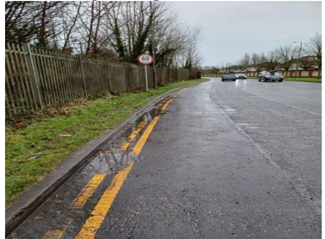
New double yellow lines on the Littlepace Distributor Road installed in late 2023.
