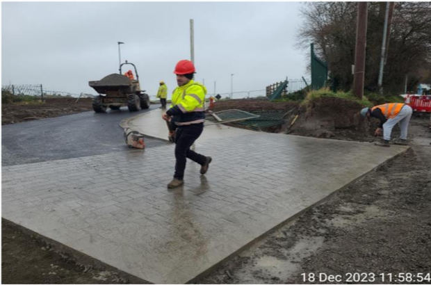
Image 9-8 Parklands entrance to Church Road South
