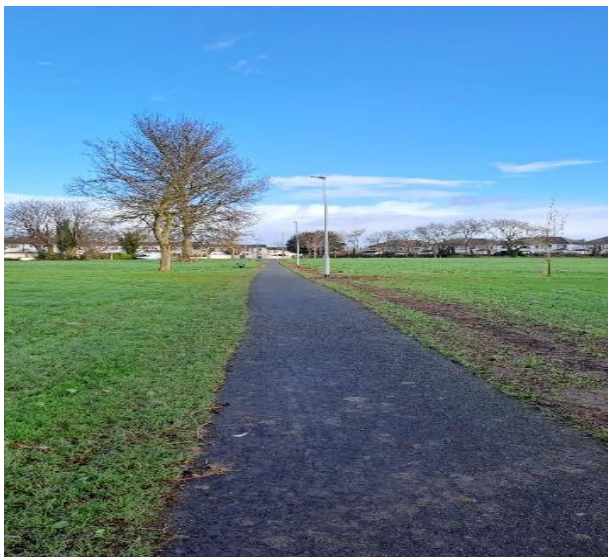
Recently installed public lighting along footpaths in public open space linking Broadmeadow and Castlefarm Estates to the Rathbeale Road Swords.
