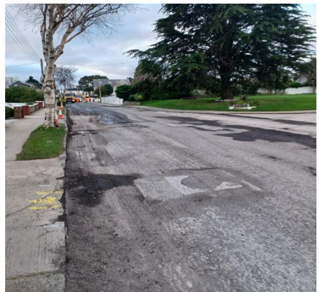
Texas Lane being planned off prior to resurfacing.
