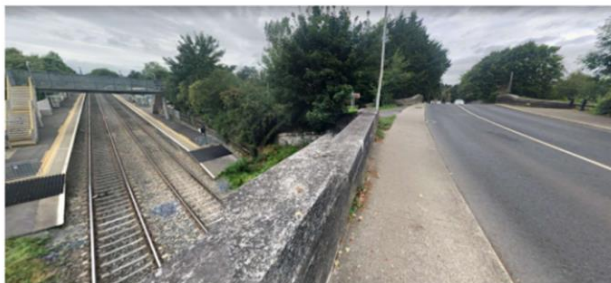
Figure 1 - View from Rail Bridge towards Granard Bridge and Blanchardstown
