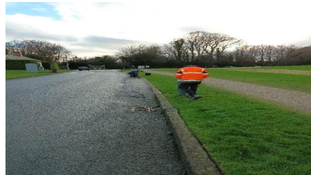
Fingal Staff Working at the Hard Edging along Main Avenue
