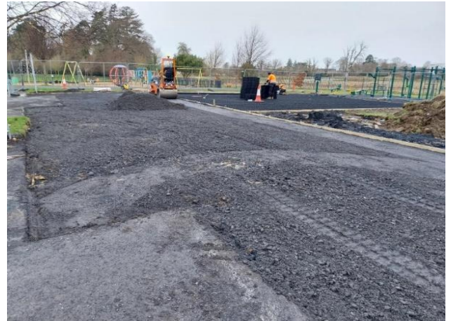
Car Park resurfacing/extension Works been carried out at Beechpark, Clonsilla.
