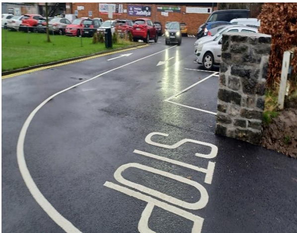
Recent Car Park marking undertaken at Verona Football Club, Blanchardstown.
