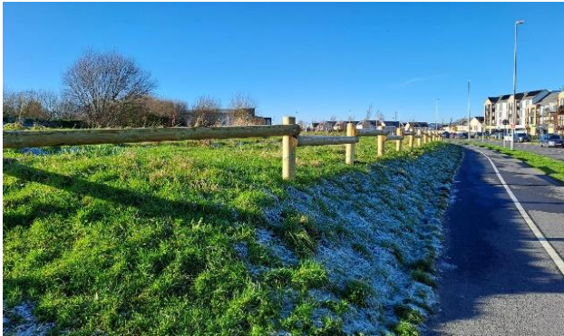
Recently installed Timber Knee Rail Boundary around Rathbeale Archaeological Park.
