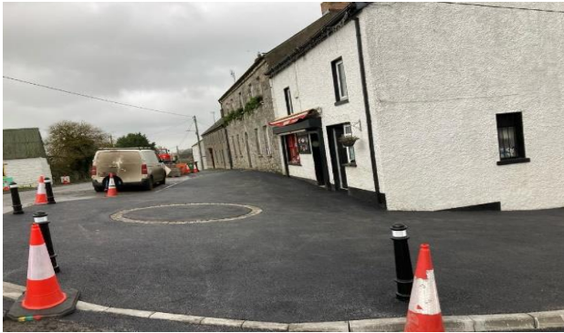
Garristown- New Kerb Build Out Garristown Main Street
