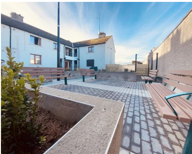
4 Rear Area - After Upgrade with Seating and Raised Beds
