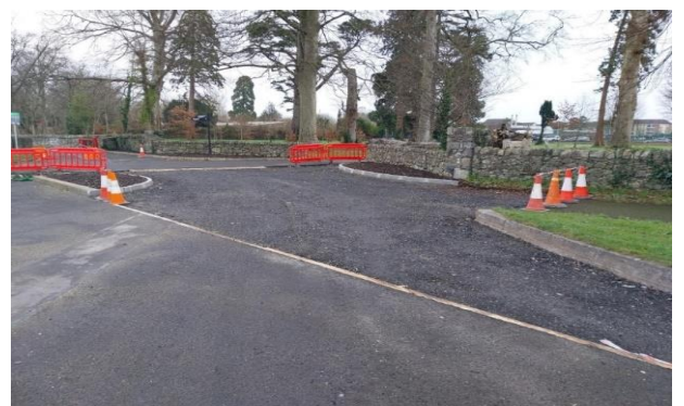
Footpath widening works been carried out at Millennium Park, Blanchardstown.
