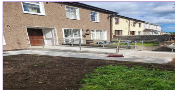
Installation of Level Access Shower and ramp at Council property
