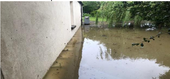
Flooding around house along the Moyne Road
