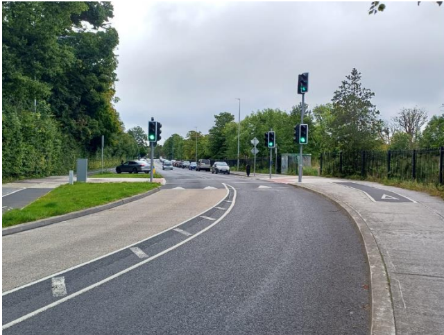
New pedestrian crossing in Clonsilla (facing towards Clonsilla train station)
