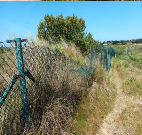
Repair to dune fencing at Portmarnock Beach.
