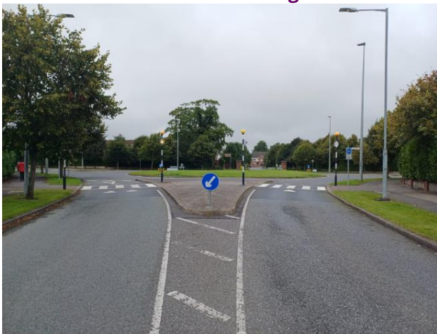
Pedestrian crossing on Main Street, Ongar after being relined.
