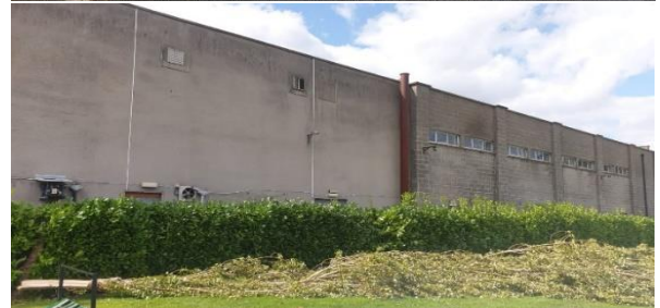
Storm betty aftermath at our burial grounds Balgriffin Fingal clean-up operation in action.
