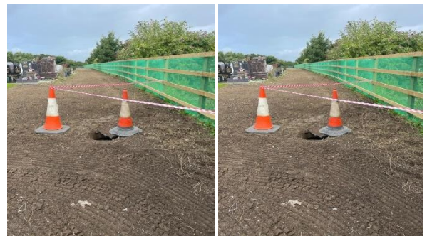
New fencing and grounds work replacement of old chamber covers.
