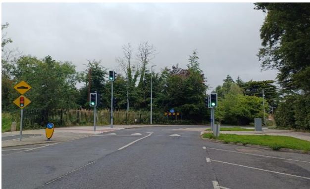
New pedestrian crossing in Clonsilla (facing away Clonsilla train station)
