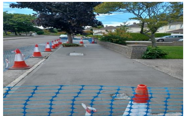
Footpaths Replaced Carrickbrack Heath Sutton
