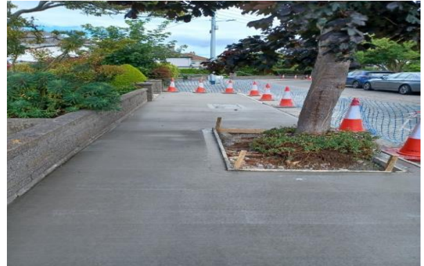
Footpaths Replaced Stapolin Baldoyle
