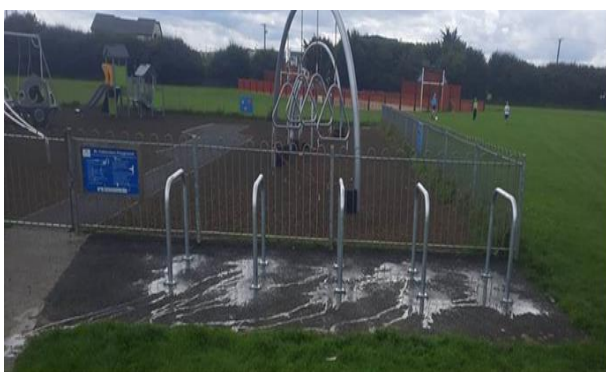
Recently installed Bicycle Stands at St. Catherine's Playground, Rush, Co. Dublin
