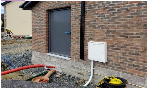
Checking depth of services in a housing development in Dublin 15.
