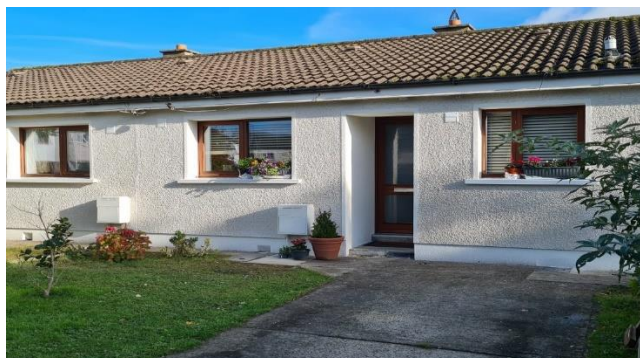
External wall insulation at retrofitted property
