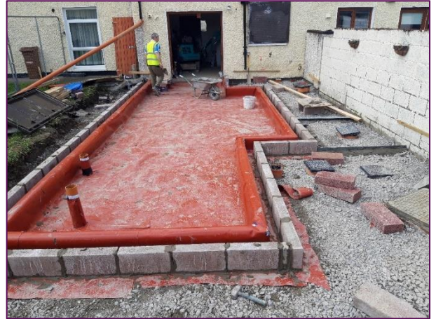
DPG extension works underway at a Council tenancy in Dublin 15
