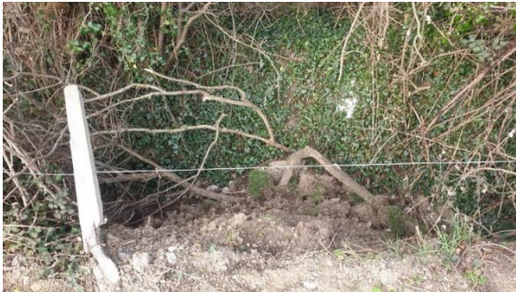
Preparation works underway for the installation of Anti Climb Fencing
