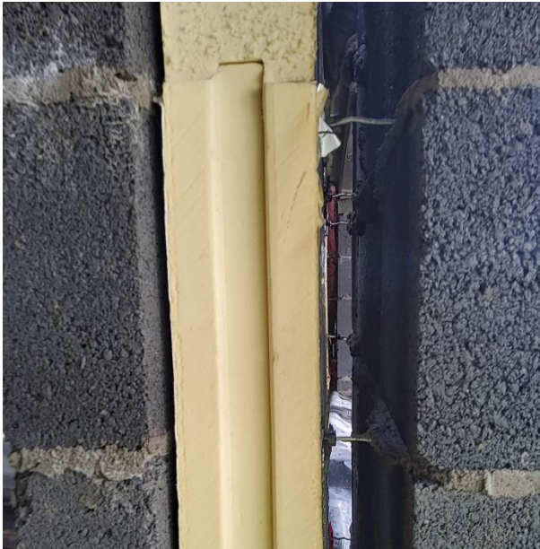
Checking Insulation in a Cavity wall in a development in Balbriggan.
