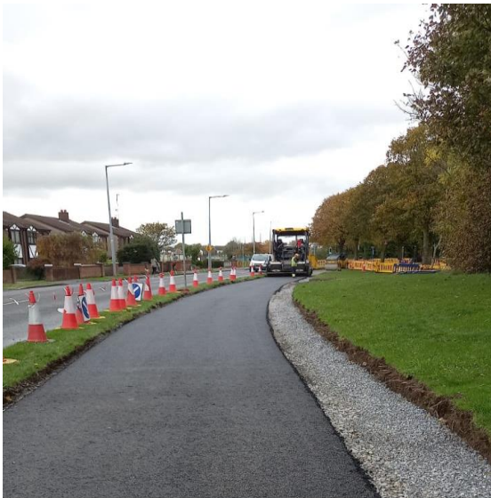
Figure 3: New two-way cycle path along Brackenstown Road
