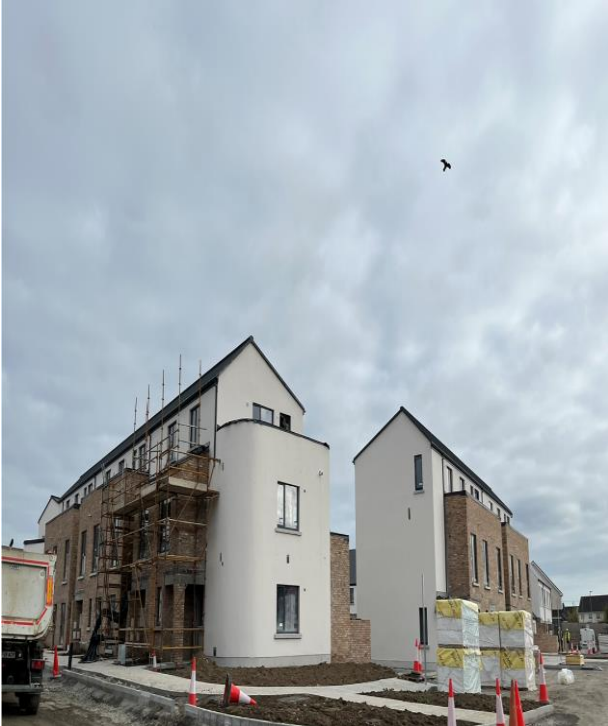
Fingal County Council construction scheme at Cappagh, Dublin11 - 69 units being built
