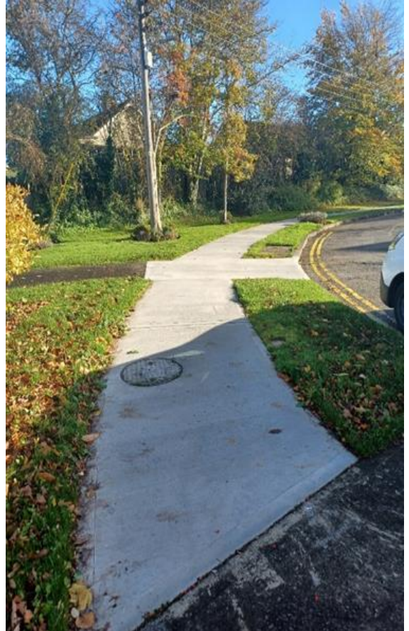
- Pavement Replacements, Ramor Park
