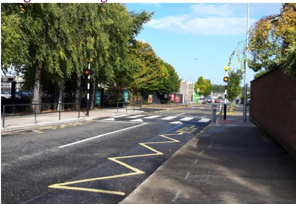
Newly constructed raised Zebra Crossing on Beechpark Avenue
