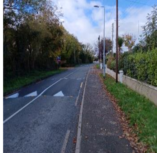
One of four ramps installed on Baskin Lane
