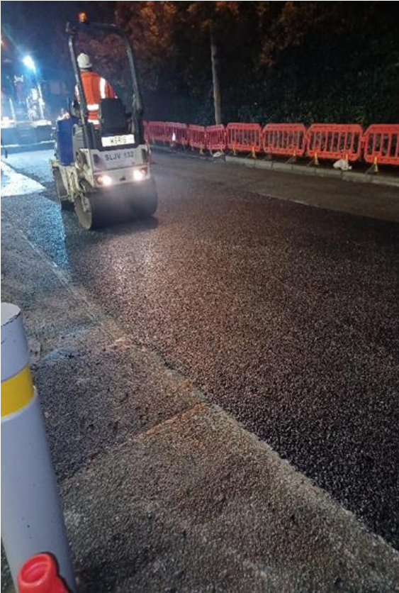
- Resurfacing Works, Coolmine Road
