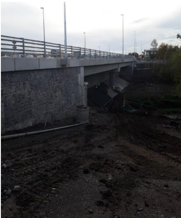
Works progressing on Snugborough Bridge over the Tolka River.
