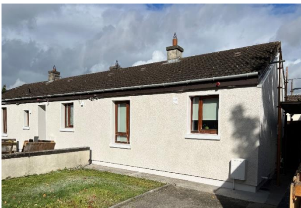
External Wall Insulation completed in Whitechapel, Clonsilla
