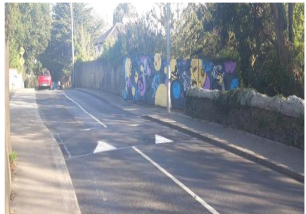
Swords – Brackenstown Road – Two speed ramps
