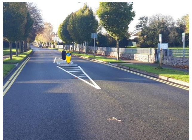
A central refuge island outside Mountview pitches in Blanchardstown
