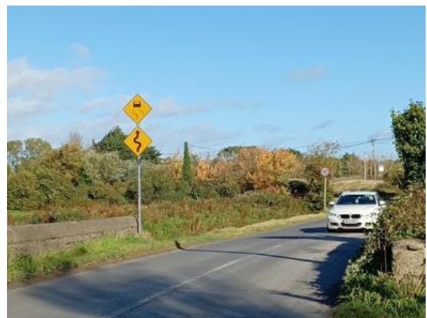
Additional warning signage on the Drumnigh Road
