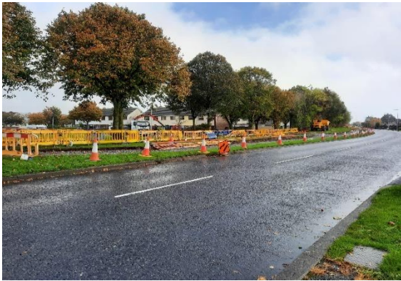
Figure 2: New two-way cycle path along Brackenstown Road
