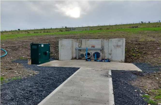
Leachate Cell Side Riser replacement works
