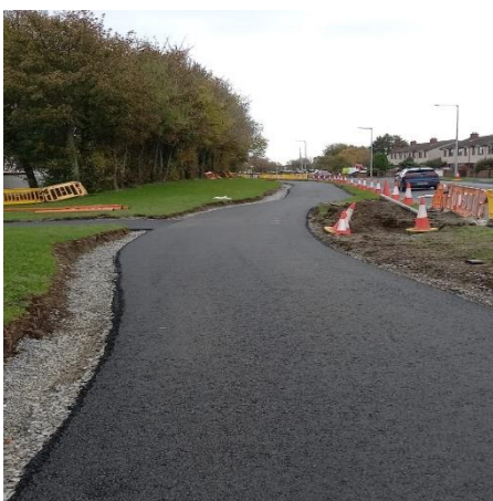
Figure 4: New two-way cycle path along Brackenstown Road
