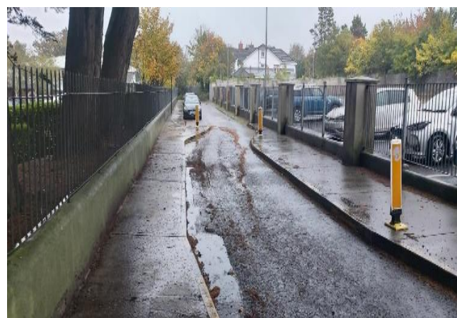
Howth Culvert Stormwater Network Upgrade
