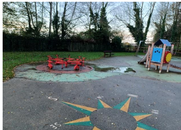
Flooding relieved with new drainage
