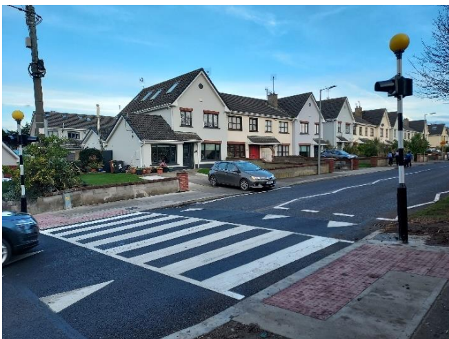
Balrothery- New Raised Zebra Crossing at Rosepark/ Coach Road
