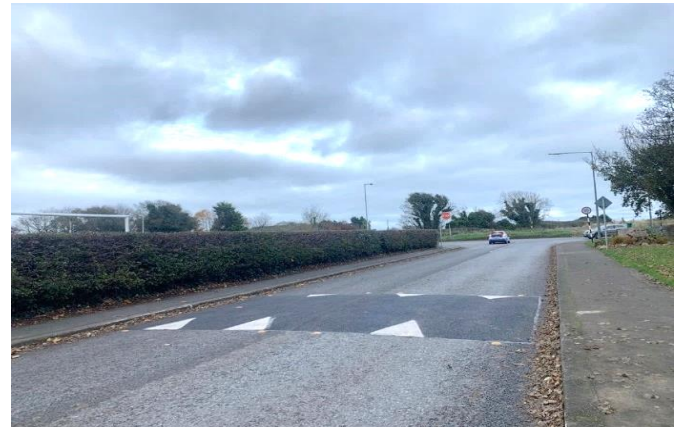
Rush- New traffic calming ramps at St Catherine's Estate for traffic calming in the vicinity of St Catherine's National School.
