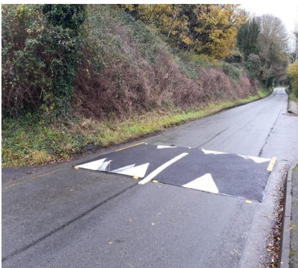
Newly constructed ramps on Lower Road
