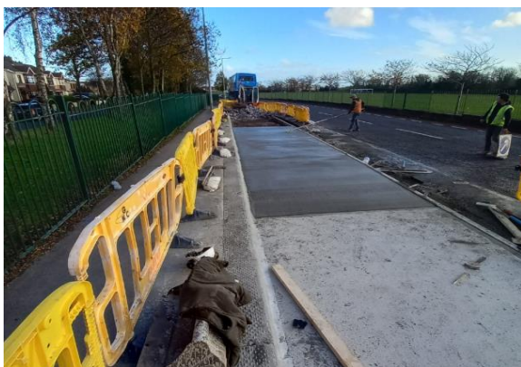
Figure 2: Replacement of broken concrete along bus layby on Brackenstown Road
