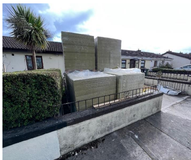
External insulation delivery on site
