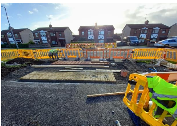
Figure 1: Zebra Crossing Brackenstown Road
