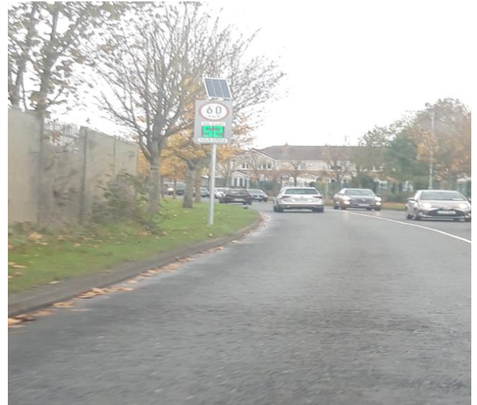
A newly installed Solar Powered Speed sign was installed on the L-3025 (Littlepace) in November.
