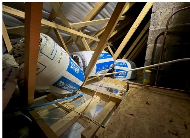
Attic insulation in progress
