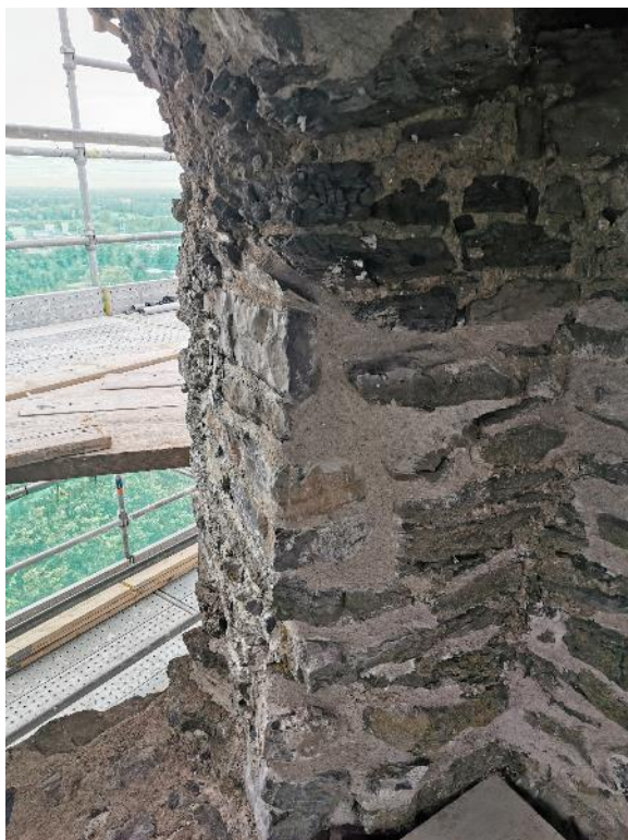
The NE corner after conservation
