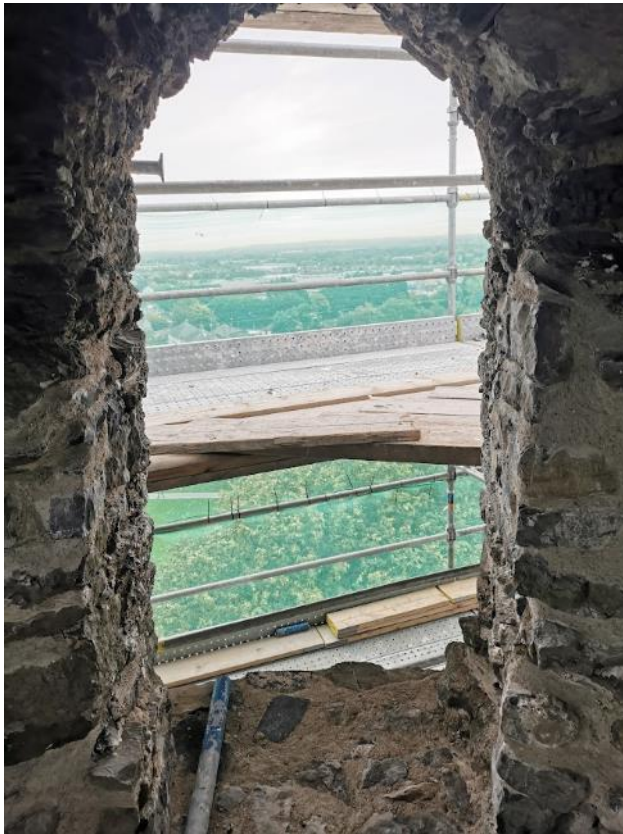
Looking at the North window from the interior of the tower
