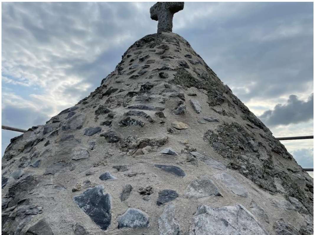
Completed work on the roof
