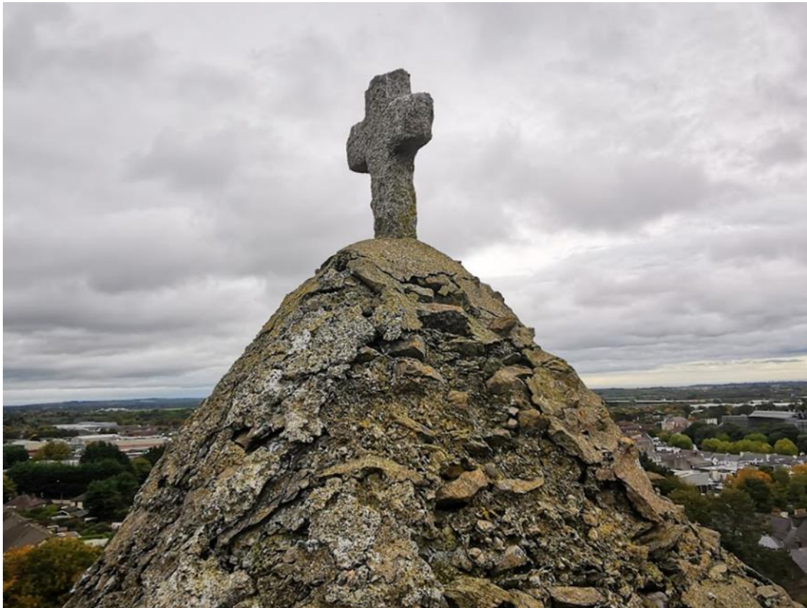
Round tower roof prior to conservation
