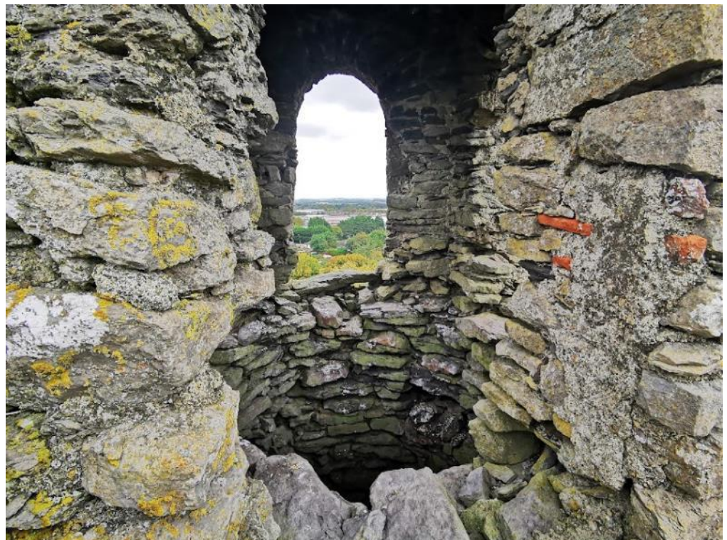
View of the north window prior to conservation works
