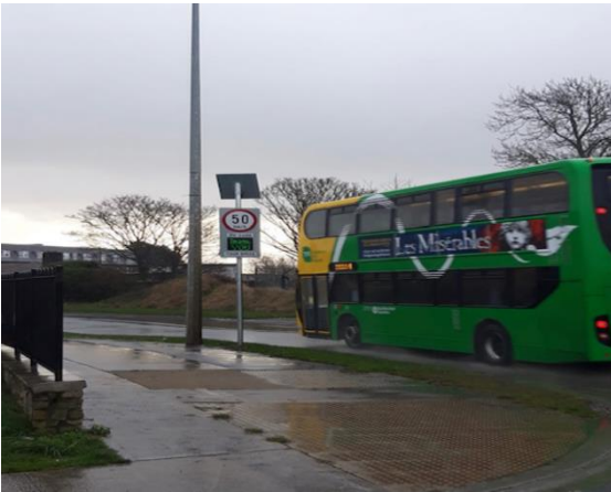
The sign on Beechpark Avenue/Auburn Avenue required replacing
