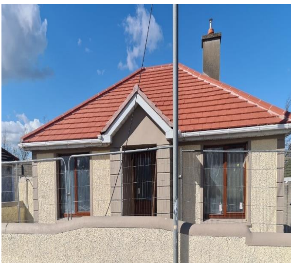
Group Housing Scheme Refurbishment Works
