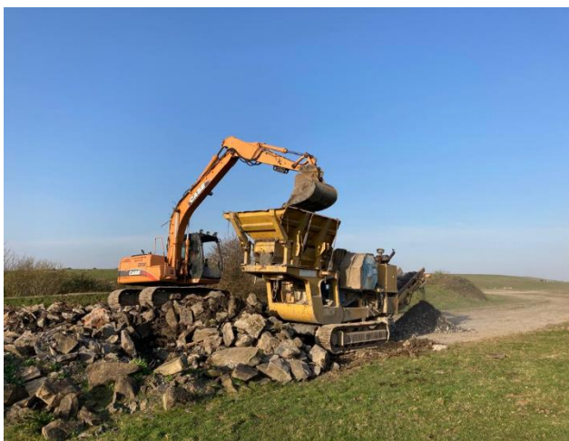
Photograph 1: Excavator feeding the Crusher with large rocks sourced from the landfill
