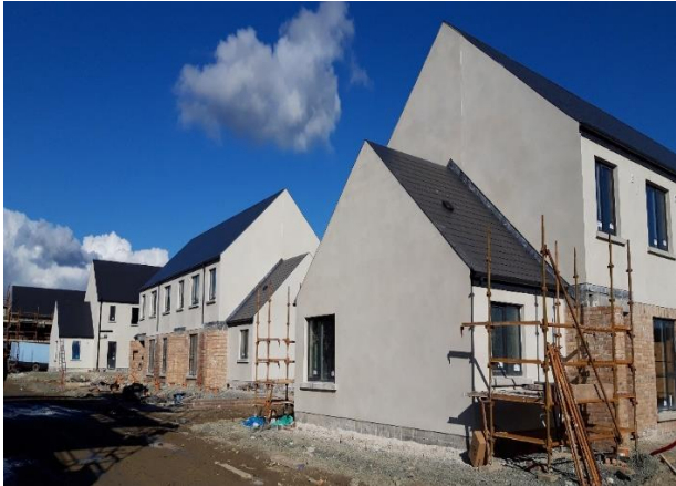
Fingal County Council construction scheme at Cappagh, Dublin11 - 69 units being built
