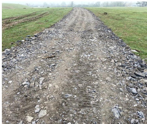
Photograph 3: The crushed stone used as a base for the internal road network.
