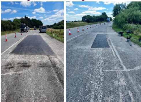
Road Patching Works on the R132 near Ministers Road Junction
