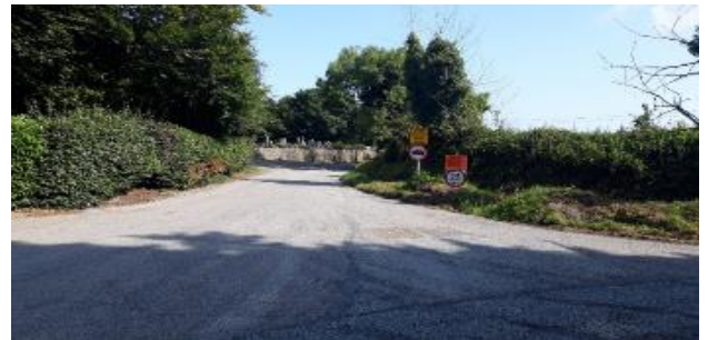
Surface dressing works at Kileek
