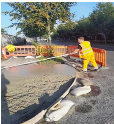
Melville Road - Footpath Repairs
