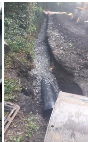
Road drainage works Corrstown
