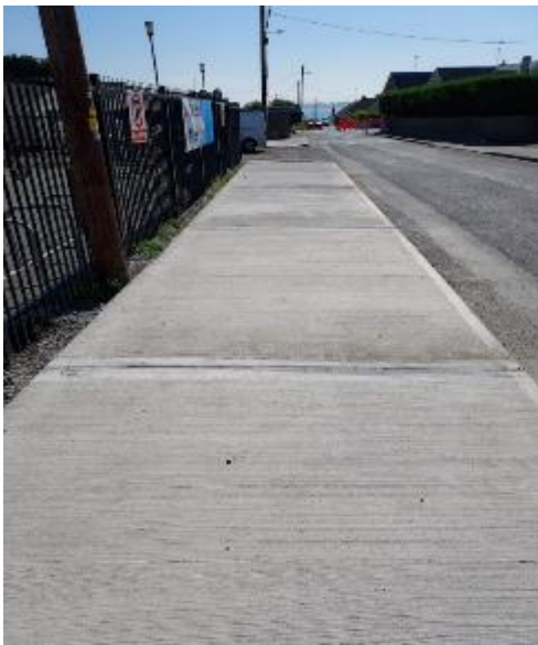
Footpath works Convent Lane Rush
