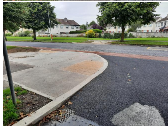
Hartstown/Huntstown Kerb Protected Cycle Lane – New Uncontrolled Crossing Points and Junction Build Outs
