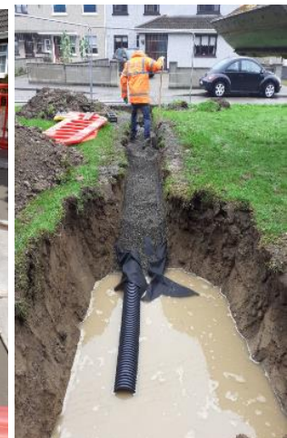
Drainage works at Derham Park Balbriggan
