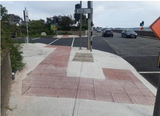
Bayside Boulevard and the Dublin Road - new pedestrian crossings completed with new updated LED signals with control system (MOVA) to be installed soon
