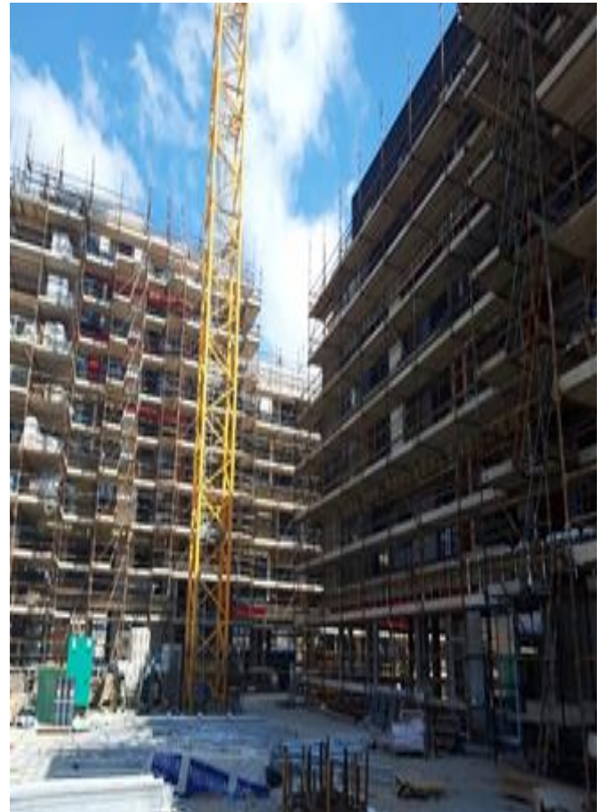
August 2021 – BC inspection of Apartments in Hansfield
