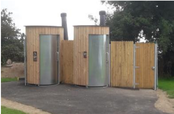
Recently installed Eco Toilets at Ardgillan Upper car Park
