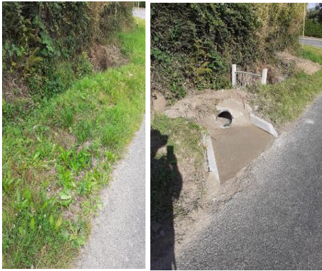
Drainage works at Flemington Road
