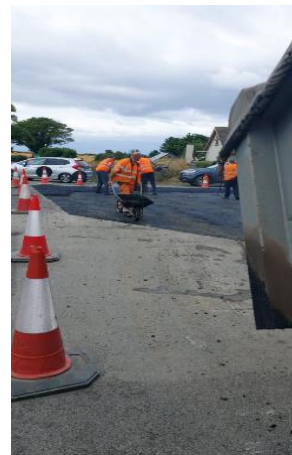
Road Improvement works
