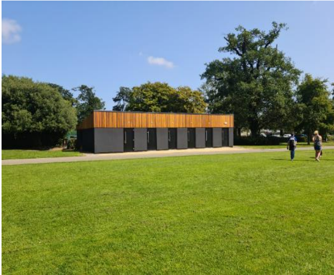
Newly installed Public Toilets at Santry Demesne
