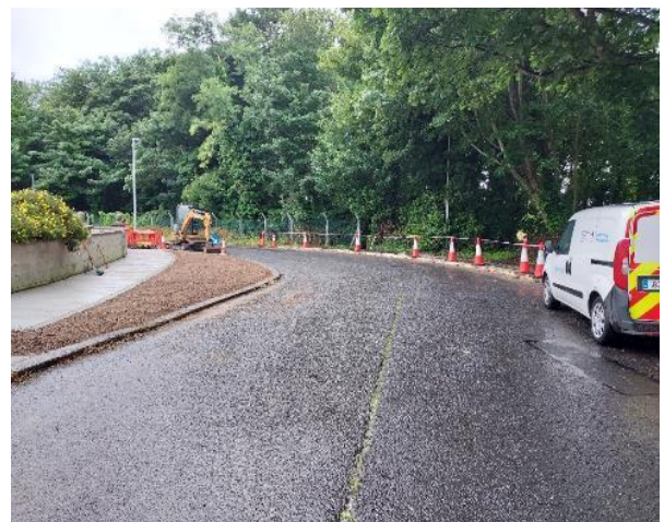
New section of footpath including new verge strip at Grace O'Malley Park
