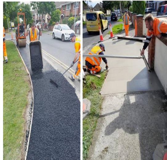
Footpath Repairs – Woodvale, Blanchardstown
