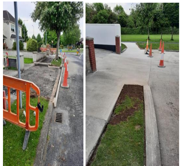
Footpath Repairs - Sycamore, Castleknock.
