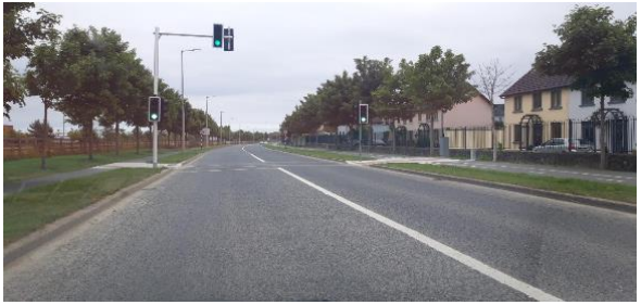
R127 at Clonrath Estate Lusk – New Signalised Pedestrian Crossing
