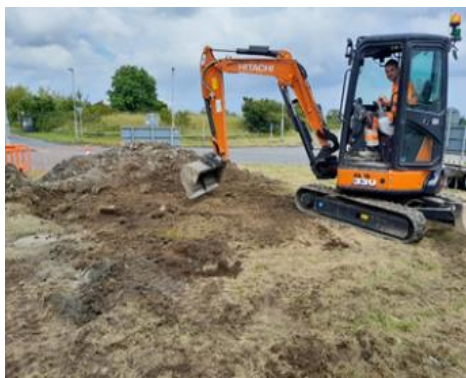
St. Margaret's Road – Drainage Works
