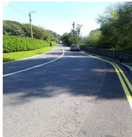
Double yellow lines added to a 90-degree bend on Barnhill Road in Lucan
