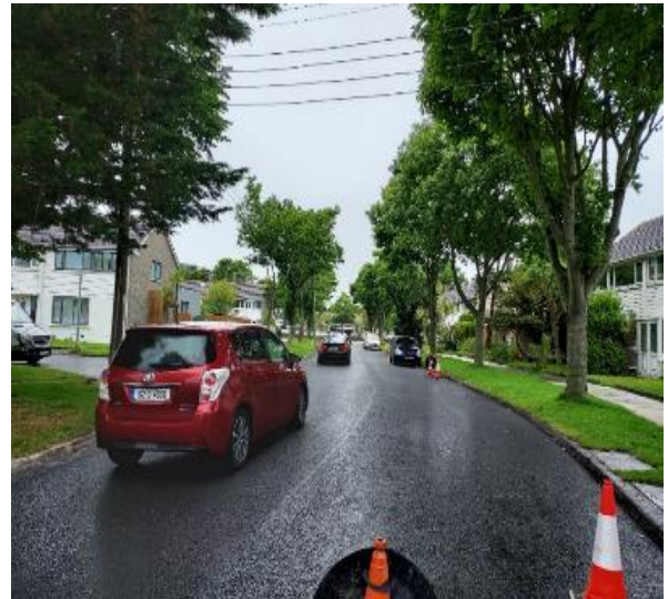
Bayside Boulevard after the final phase of resurfacing works
