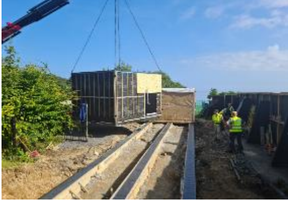
Ardgillan Playground Toilet Refurbishment - Site preparation and arrival of units.
