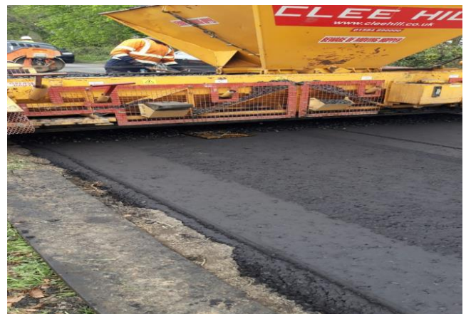
Chip spreading to the HRA Mat (note quality control tray test).
