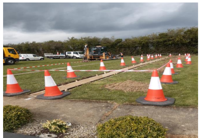
Concrete works in Rolestown Cemetery
