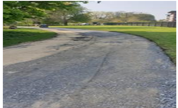
Santry Demesne – Footpath Widening
