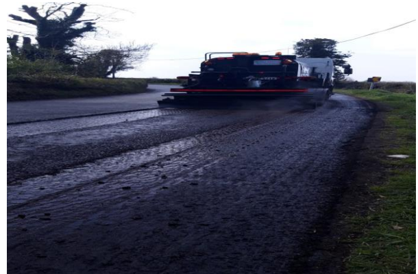
Application of the binder coat
