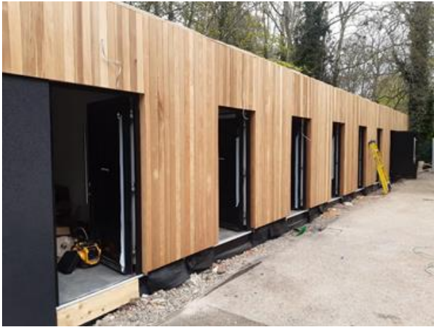
Construction of replacement toilets at Newbridge Demesne Playground
