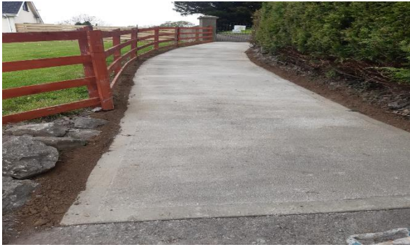
Entrance Upgrade Works to Chapelmidway
