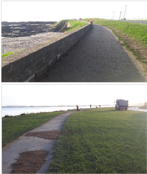
Crews working repairing various coastal walkways in the Howth Malahide area
