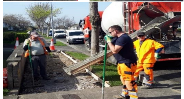
Staff constructing footpath bays in Inbhir Ide and Sonesta, Malahide.
