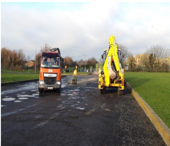
Remedial works being carried out at Paddy's Hill
