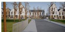
Street view towards north units
