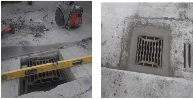
Drainage works being undertaken
