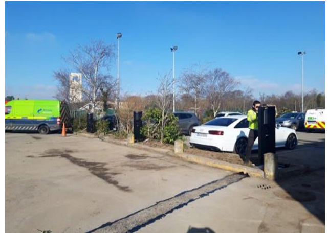
Coolmine Depot EV installation
