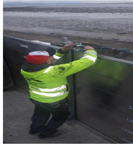
Erecting the Coastal Flood Defence System in Sutton
