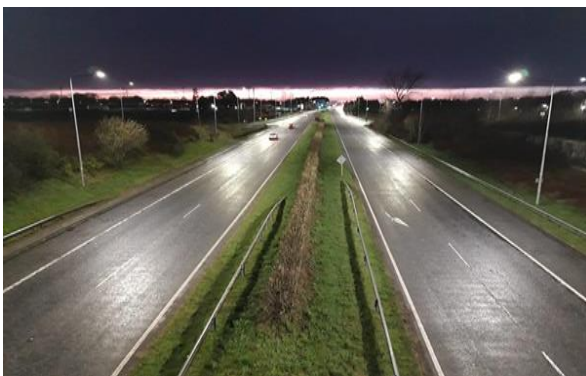
R147 Navan Road Castleknock LED upgrade
