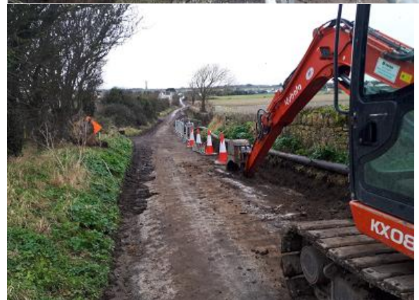
Loughshinny Foul Sewer Rising Mains on Mine Road progressing well.
