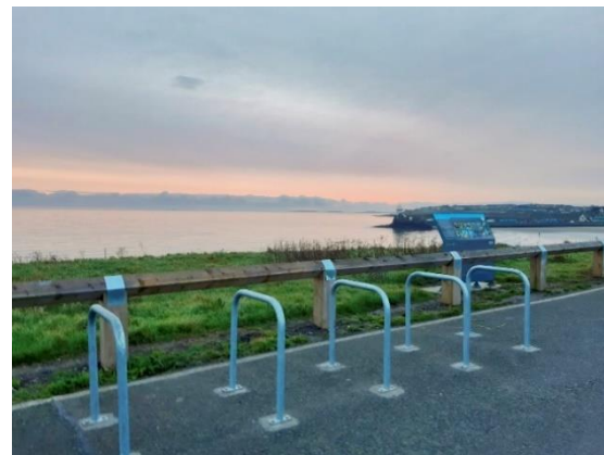
Bike Racks recently installed at Balbriggan beach
