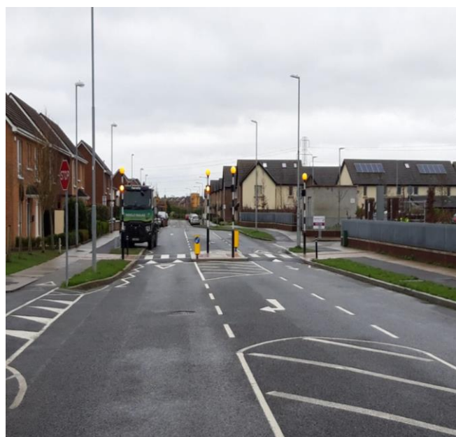
Barnwell Road, Ongar, Dublin 15. New Signalised Zebra Crossing
