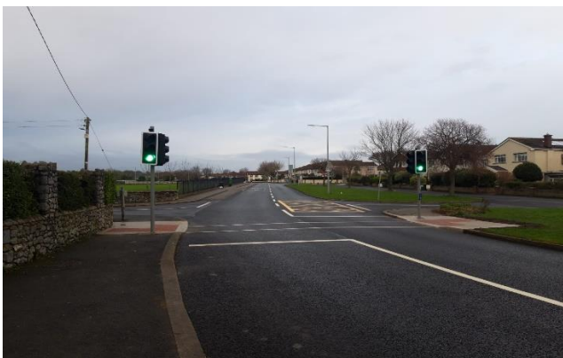
Recently completed upgrade at Carrickhill Road Lower, adjacent to the Portmarnock Community School
