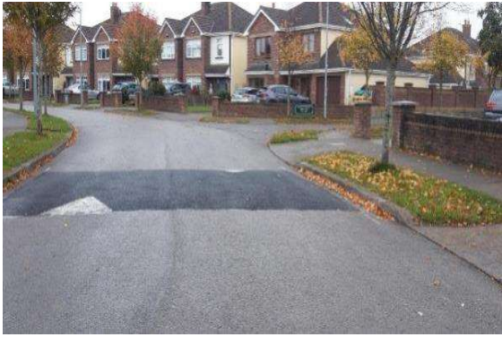
Newly installed Ramp - Carr's Mill, Donabate
