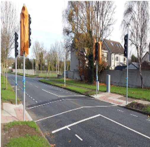
Newly installed Toucan Crossing – St. Cronan’s Avenue, Swords - Awaiting ESB supply
