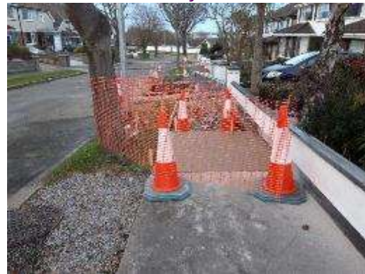
Footpath replacement works presently under construction in Biscayne Malahide
