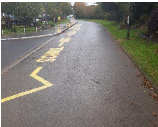
Balscadden - St Benignus NS, - New School Road Lining.
