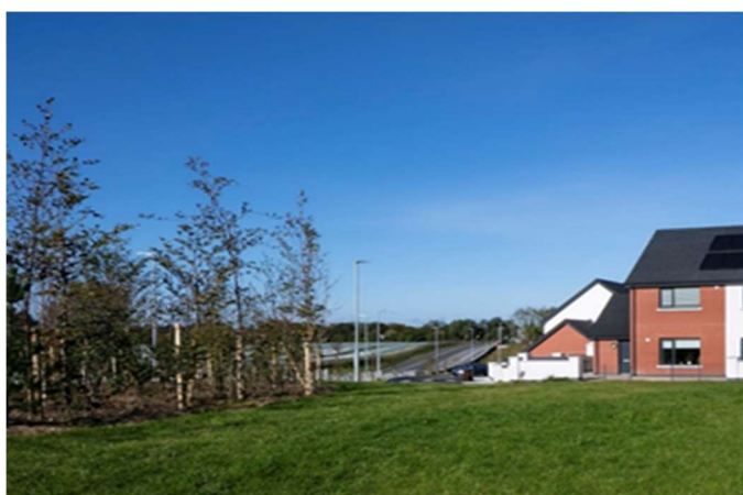
Holymount Estate, Rathbeale Road, Swords. Completed in 2020, all 24 units have a BER rating of A2 and achieved NZEB standards.
