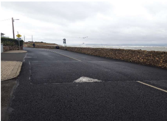
New ramp installed - Strand Road Sutton
