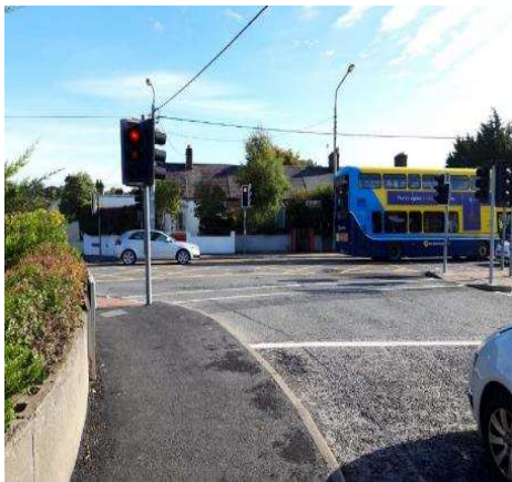
Footpath widened at Blanchardstown Main Street/Clonsilla Road junction completed in November.
