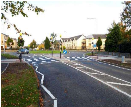
Newly installed Signalised Zebra Crossing – Diswellstown, Dublin 15 -- Awaiting ESB supply
