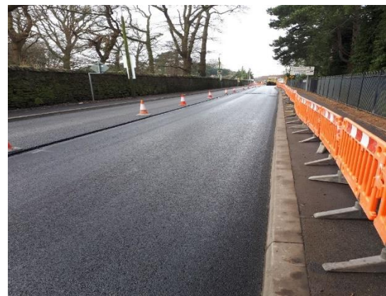
R806 Castleknock Road Resurfacing Works
