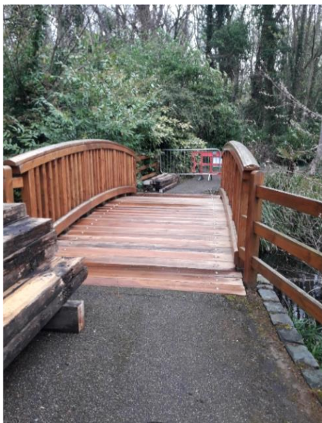
Bridge Restoration at West Lawn, Malahide
