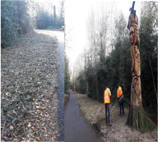
Footpath improvement works
