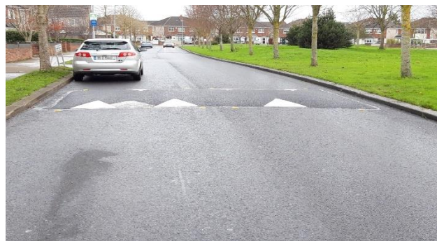
Completed ramp in Dublin 15
