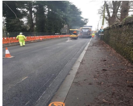
Road Resurfacing Works
