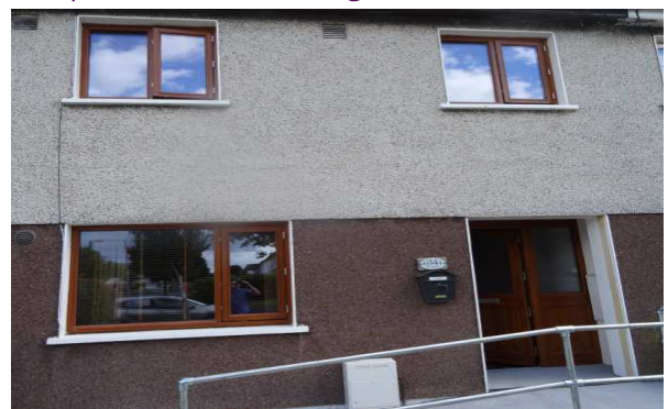
Example of Window & Door Replacement in Dublin 15
