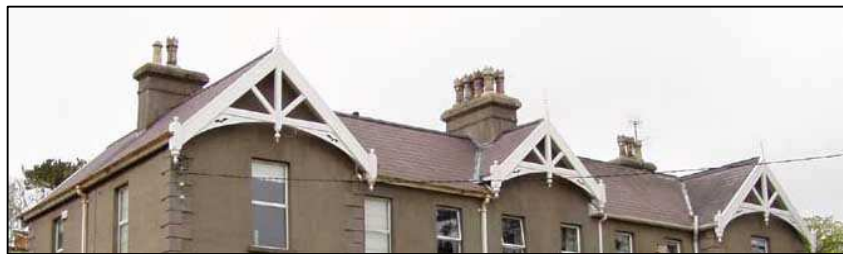
Fig. 8 Pitched slate roofs with breakfront gables & central section
