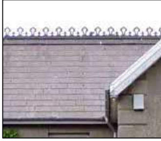
Fig. 9 Cast iron cresting
