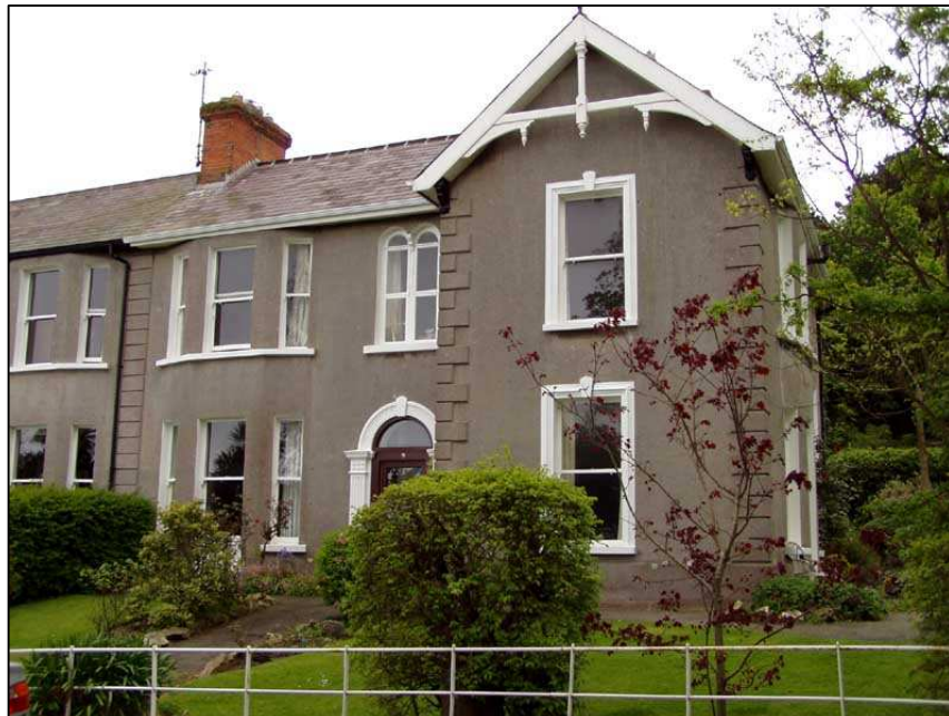
Fig. 16 No. 9 Nashville Park is part of the terrace of houses and so has irregular quoins to gable ends, regular quoins separating it from No. 10, up-and-down timber sash windows, canted bay windows, double window, and decorative front door surround
