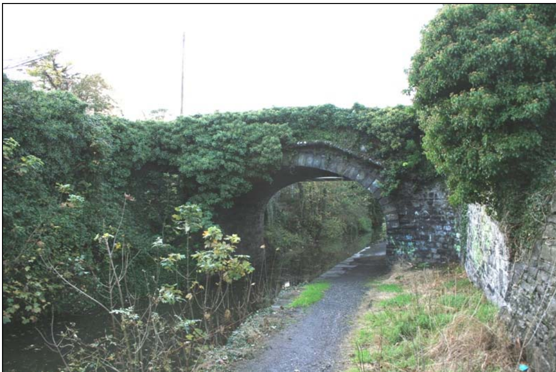
Plate 2: East elevation of Callaghan Bridge (Photo Reference: FHBS-14-BH-02)
