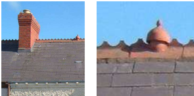
Figs.9 & 10 No. 24 Hampton St roof and terracotta air vent details
